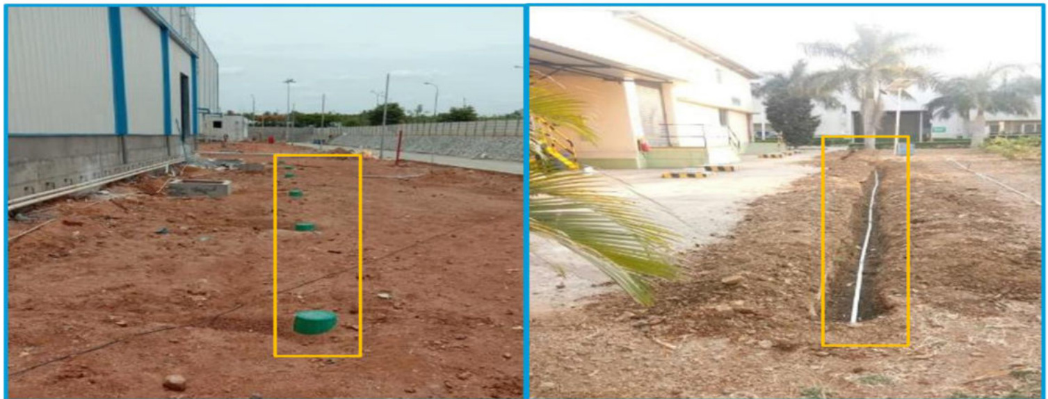
Type A & Type B Earthing Electrode
